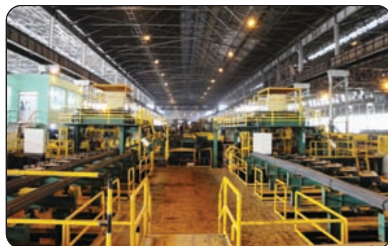
Bar Rod Bundling and Packaging Automation “Right from Cold Shear to Rail Wagon Loading”
